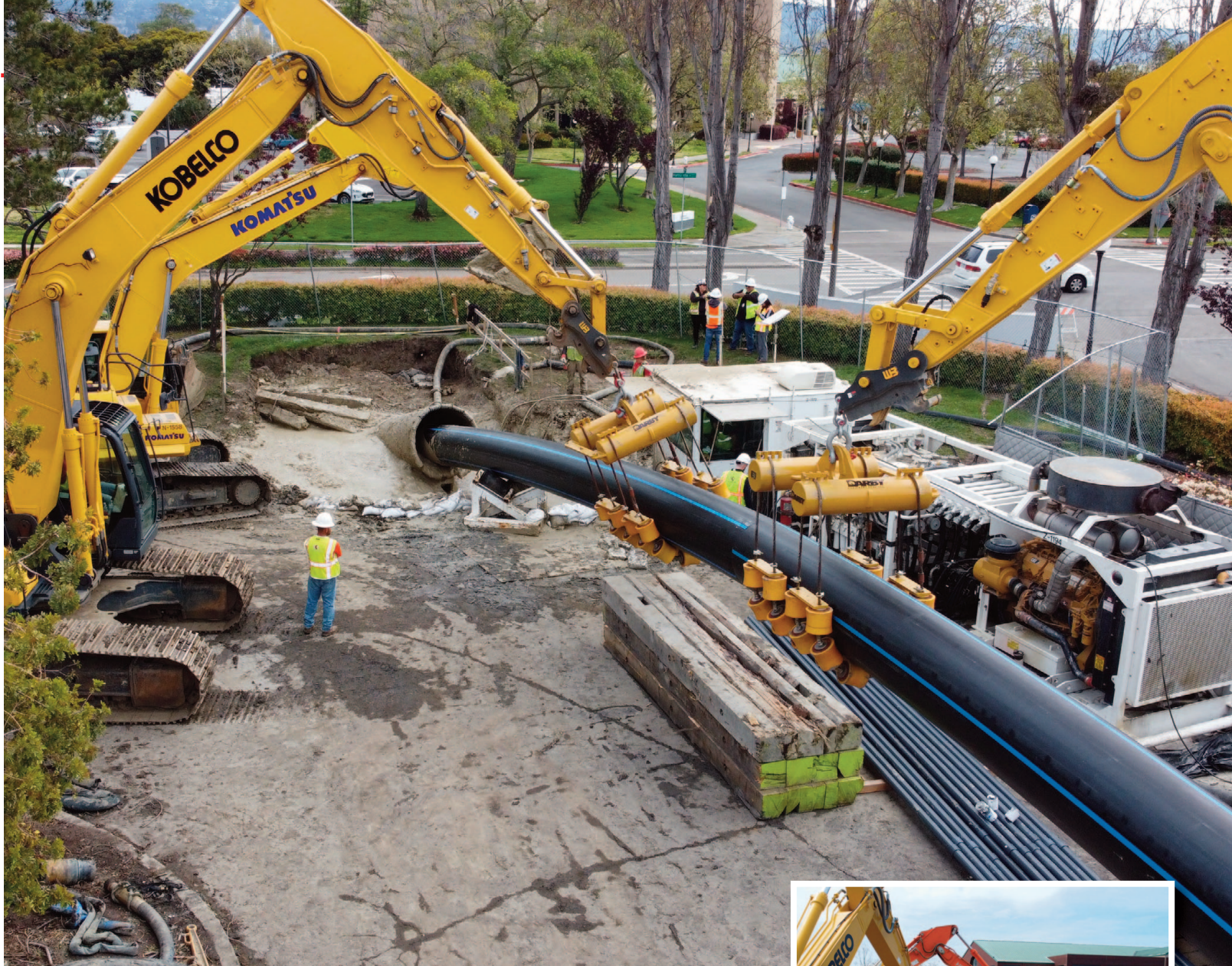
Figure 1. Steel, HDPE and FPVC pipe all elastically bend to adhere to above-ground curvature
