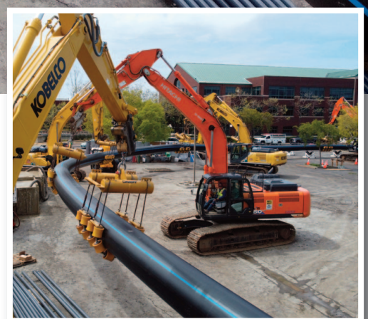
Figure 2. HDPE can turn a much tighter corner than other pipe materials
